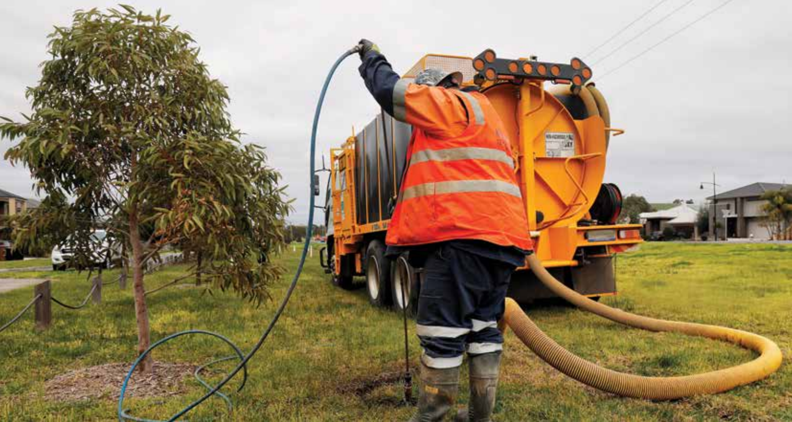
Image above: construction work
