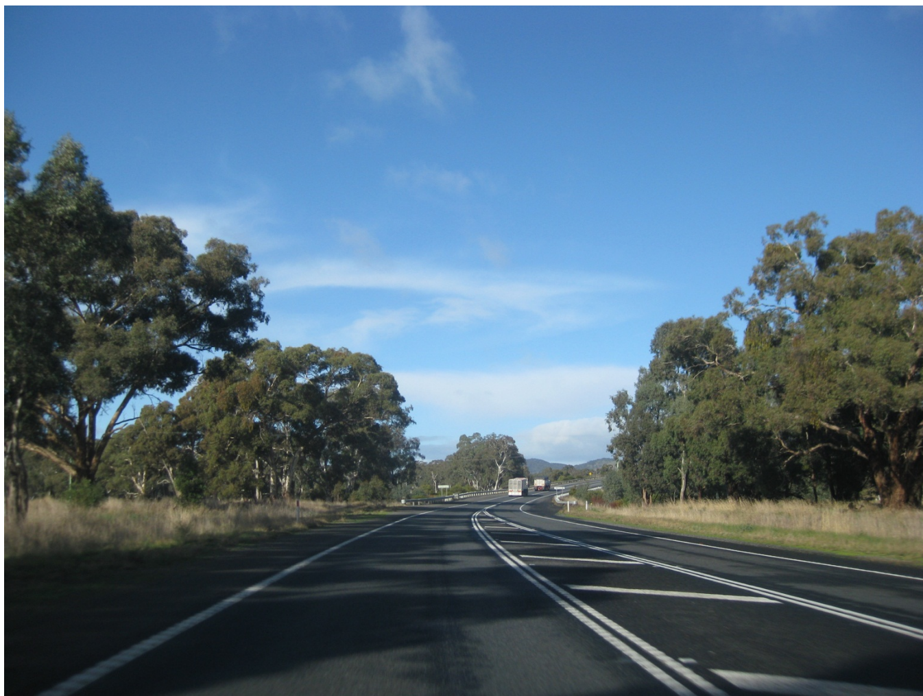
Armstrong Deviation, looking south
