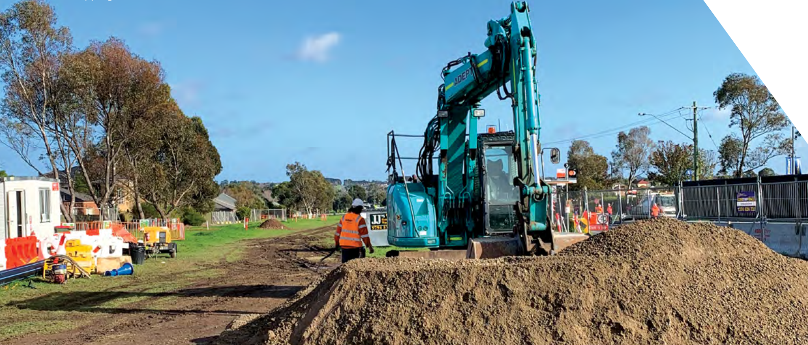
Soil stripping on O'Shea Road
